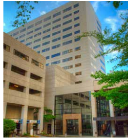
Elmer J. Nordstrom Medical Tower 1229 Madison Street, Seattle
